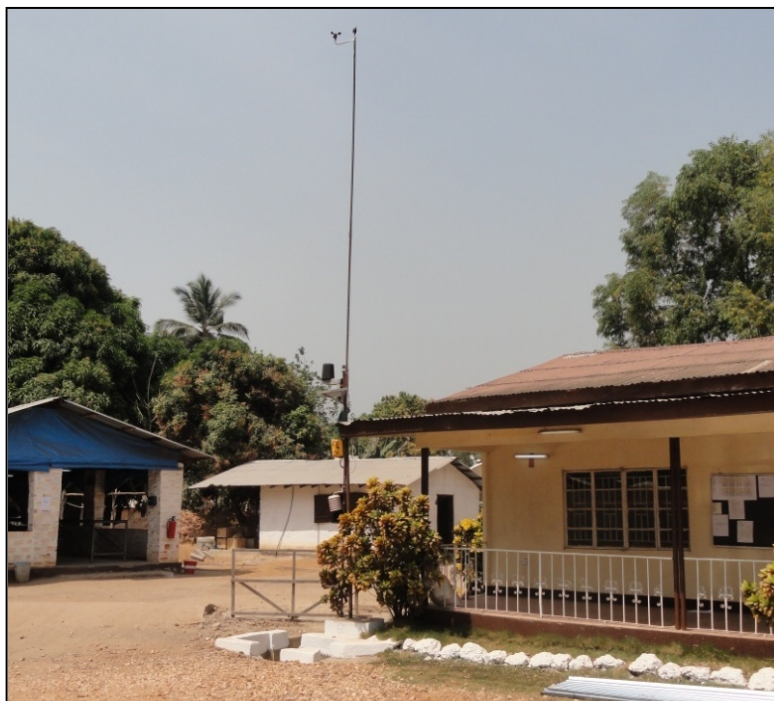
Figure 5.4: Automatic meteorological station at the MIOL site office
